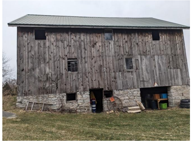
Red Barn - long elevation showing stone foundation/open lower-level areas and existing windows/openings.
