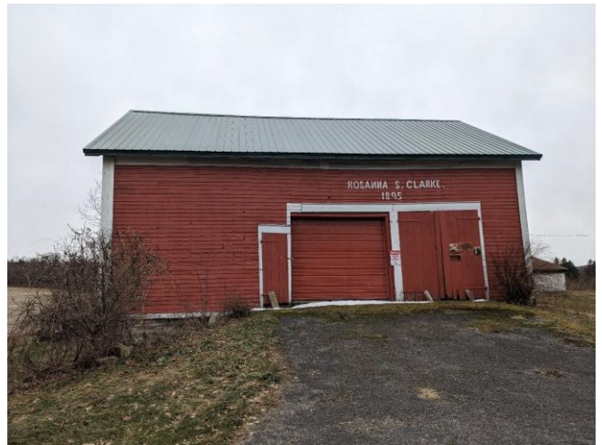
Red Barn - opposite end elevation and existing door/opening configuration.
