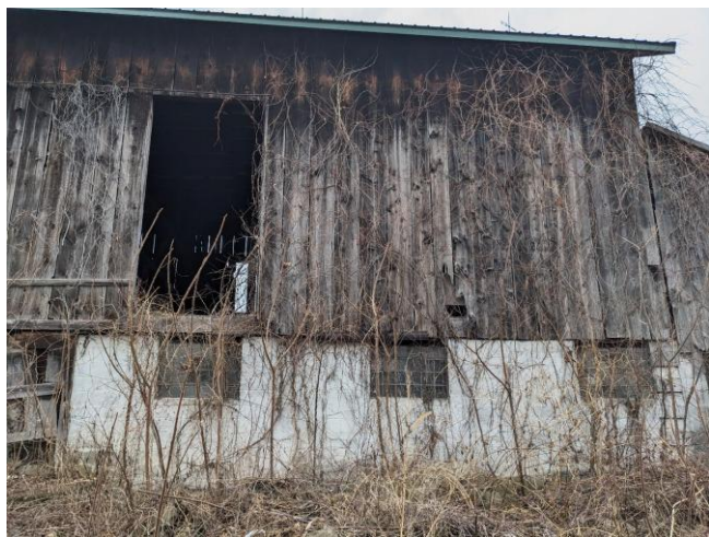
Big Barn - exterior opening and lower wall/foundation area; proposer should inspect framing, opening, envelope, and access conditions.
