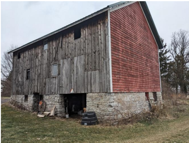
Red Barn - oblique exterior view showing stone foundation and existing siding/openings.
